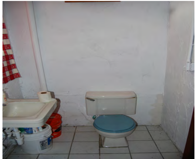
Normal Rest Room in Building
